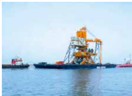
Ship unloader in Qatar
