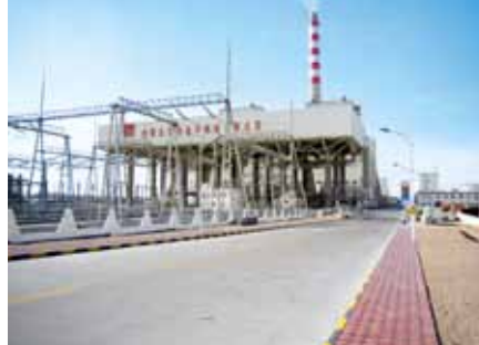
2 x 330 MW fossile fuel power plant, Jinneng, Inner Mongolia, PRC
