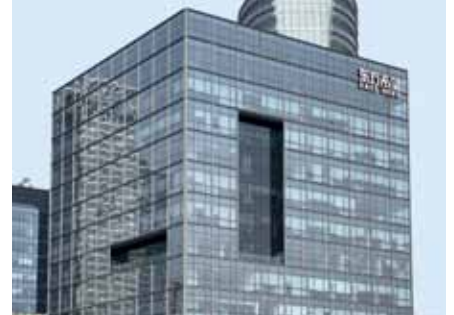
Helbling Representative Office, Shanghai, China
