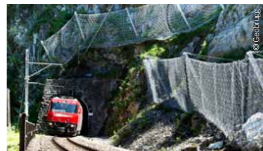
Rock fall simulations allow for optimal dimensioning of Geobrugg's rock fall barrier system RXE.
