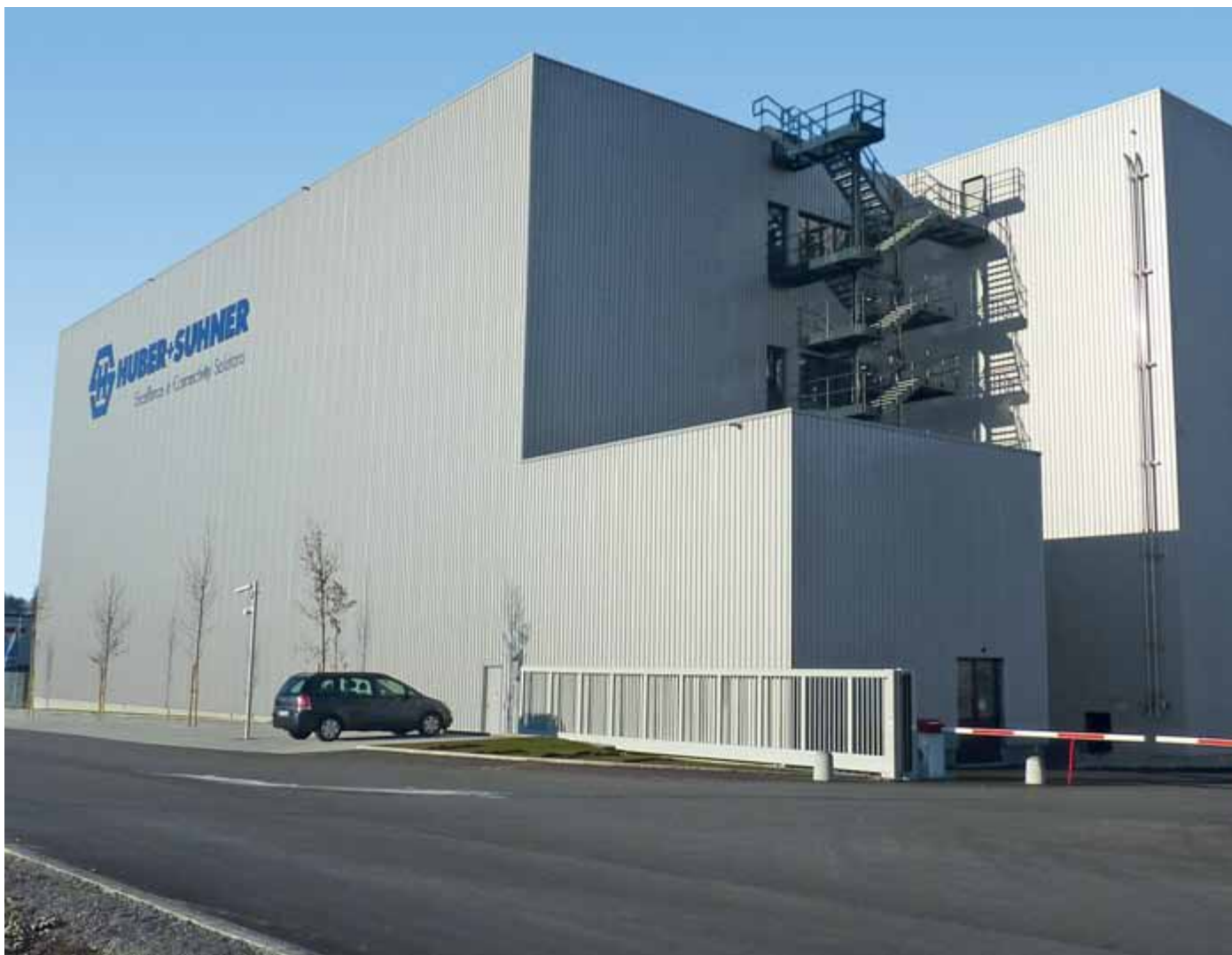
New construction of a mixing facility for Huber+Suhner in Pfäffikon near Zurich
