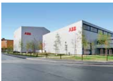
New construction of ABB manufacturing facility and laboratory building for high voltage switch gear; Helbling Beratung + Bauplanung planned the entire building technology
