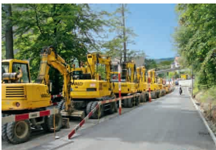
Dolderstrasse Zurich: road rehabilitation operations
