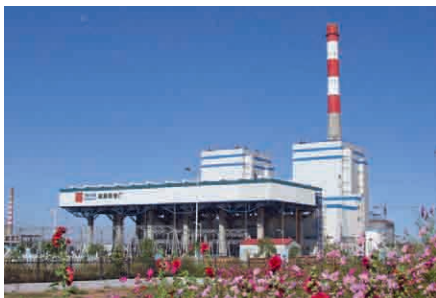
The newly built Xilinhaote thermal power plant (2x300 MW) in China prior to initiation
