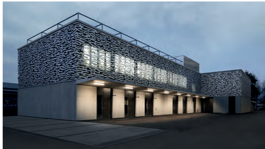
EAWAG: General planning: Refurbishment/new build of a laboratory building with MINERGIE-P-ECO certification
