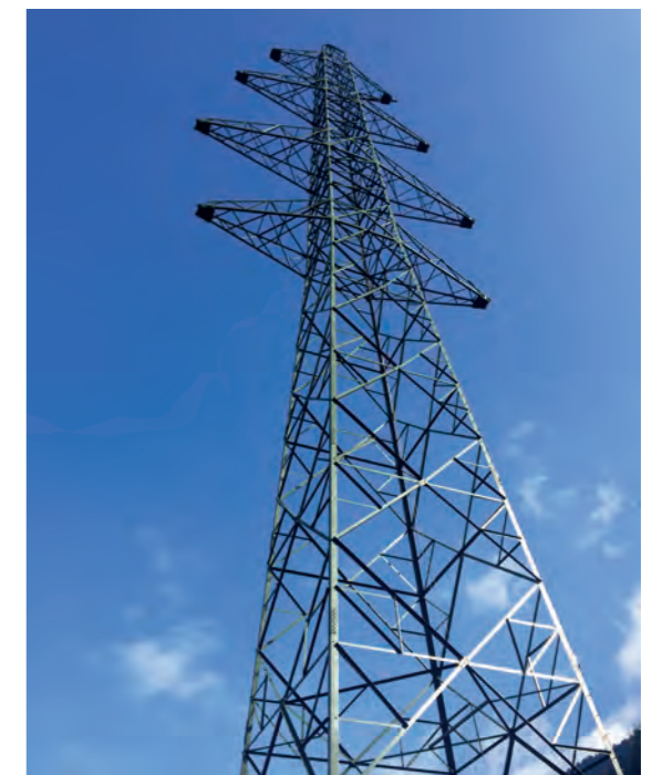
swissgrid: support for strategic purchasing New build 380kV power line Châtelard-Bätiaz
